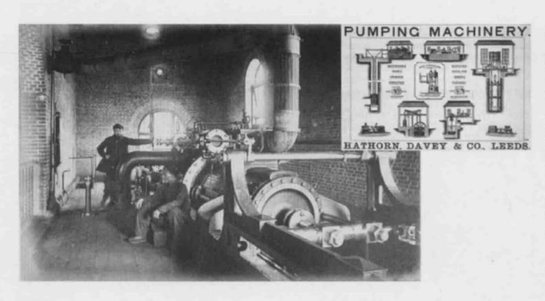
One of the steam-powered water pumping-plants, consisting of a Davey's differential engine with two separate 50 inch and 30 inch cylinders. These operated the lifting pumps in the mine shafts to prevent them from flooding. These engines were imported from England. Standing on the left is believed to be R. Burnett.
