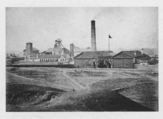
A view of the first coal mine at Tongshan shortly after boring the first two shafts and the erecting the winding gear. The tall square chimney belonged to the boiler plant where steam was generated to power the huge water pumps needed to prevent the mine from flooding. This steam was also used to power a 9.15m. diameter ventilating fan which could pump 3,400cu.m. of fresh air per minute into the mineshafts.
