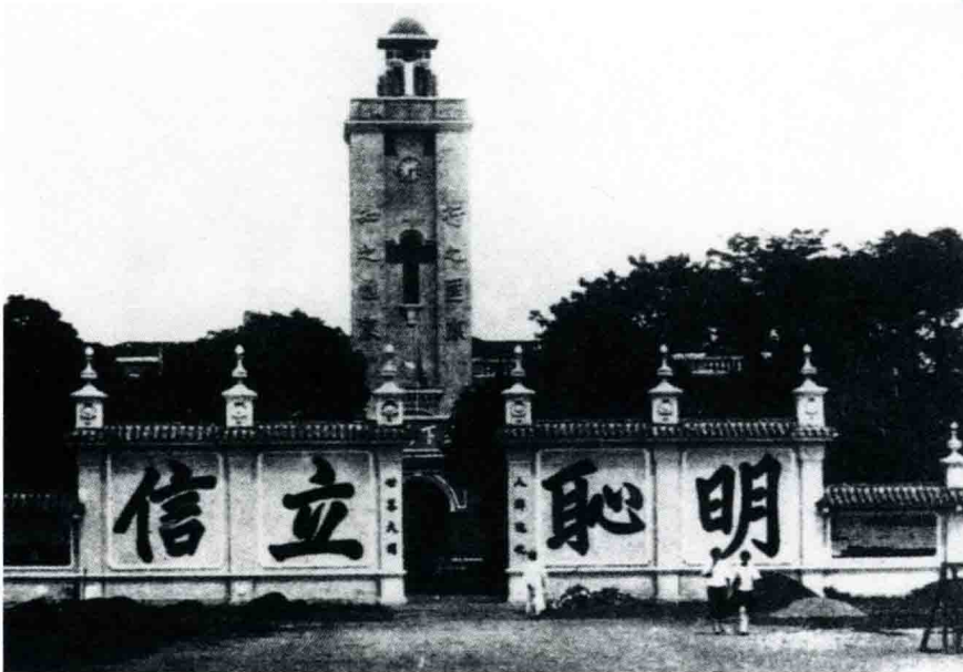
孙中山演讲三民主义的广东高等师范学校（今广州市文明路广东省博物馆内）。 The Guangzhou National Normal School (located in today's compound of Guangdong Provincial Museum), Sun Yat-sen's speeches on the Three People's Principles were made here.
